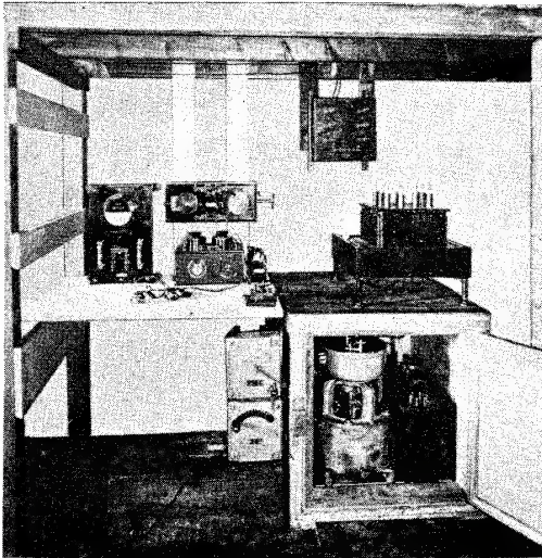
A typical ship's wireless cabin of 1912 fitted with the Marconi "1/2kW cargo set". The cabinet contains the vertical rotary converter with the disc discharger on top.
