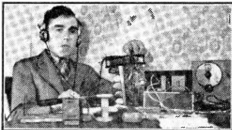
R. Ablett repairing a "38" transceiver.
