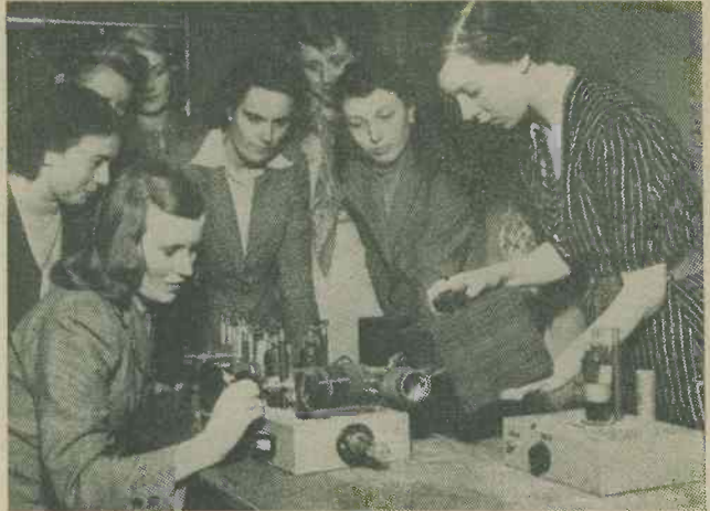
Women and girls are now being trained as radio operators by the B.B.C. Our illustration shows students being taught the principles of transmitter operation with a small table set and wægometer.
