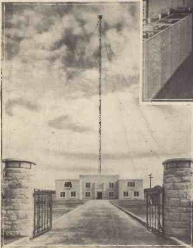
A general view of the Transmitting Hall at Burghead, and, on the left, the building and single mast aerial as seen from the entrance gates.
