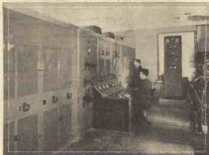
The Marconi 20 kilowatt transmitter at the Trøndelag Broadcasting Station in Norway, which has just commenced operation. This transmitter embodies the "series modulation" system.
