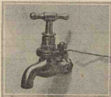
Fig. 2.—A fixing washer attached to an ordinary tap.
