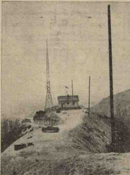
This is the U.S. Department of Commerce new aviation radio station on the high slopes of the San Gabriel Mountains at Glendale, California. From here hourly broadcasts of weather along California airways are sent out for benefit of aviators in the air.
