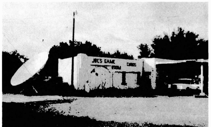
Satellite TV terminal installed at Joe's Gas Station, Nickel Creek, Texas. Photograph from John Tellick.
