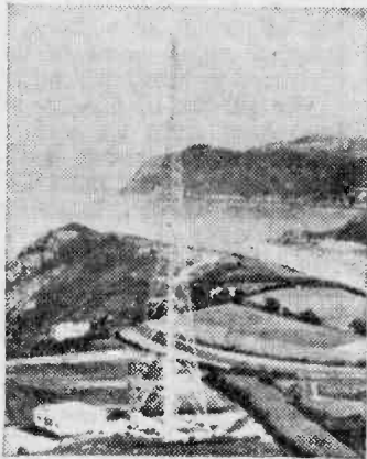
The ITA's mast at Fremont, Jersey.
