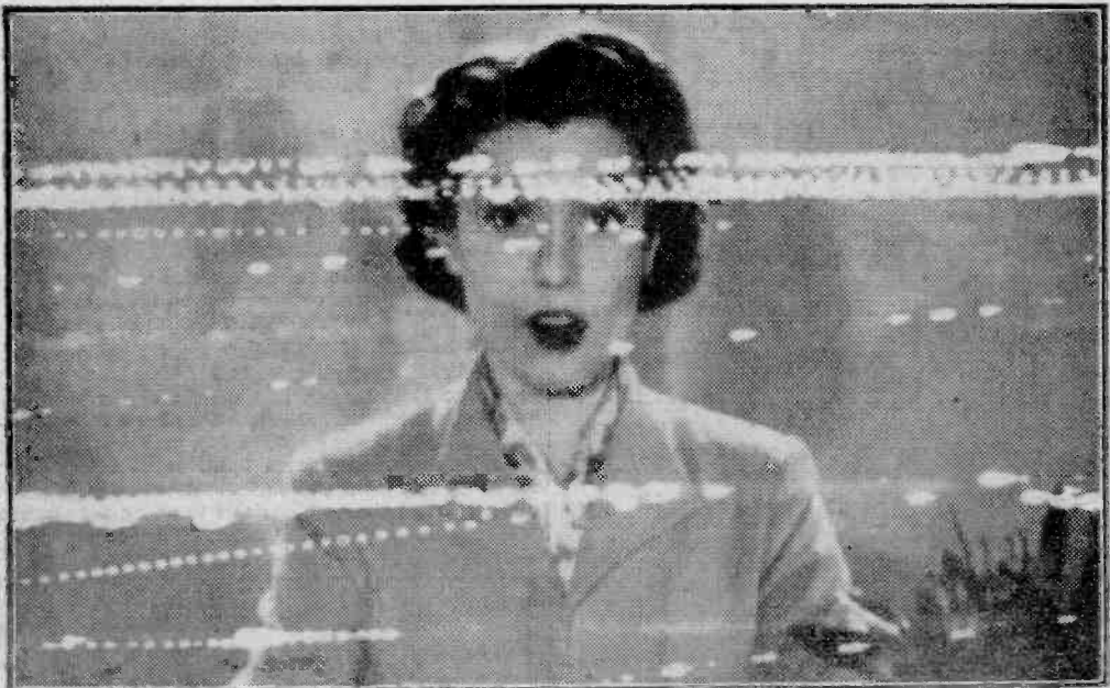
Fig. 1.—Ignition interference on a television screen.
