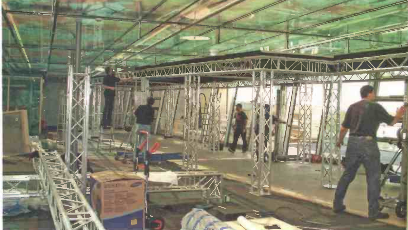
An inside shot of the studio being constructed.
