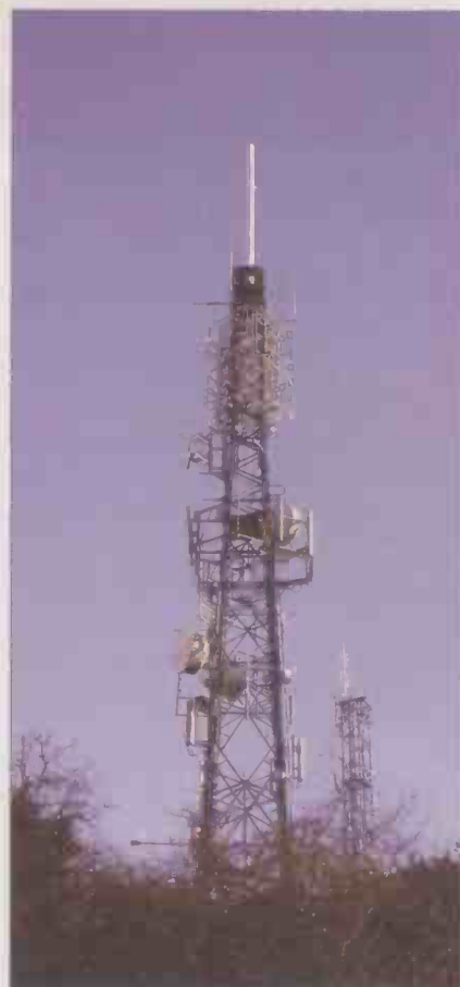
Transmitter at National Grid site, Guildford.
