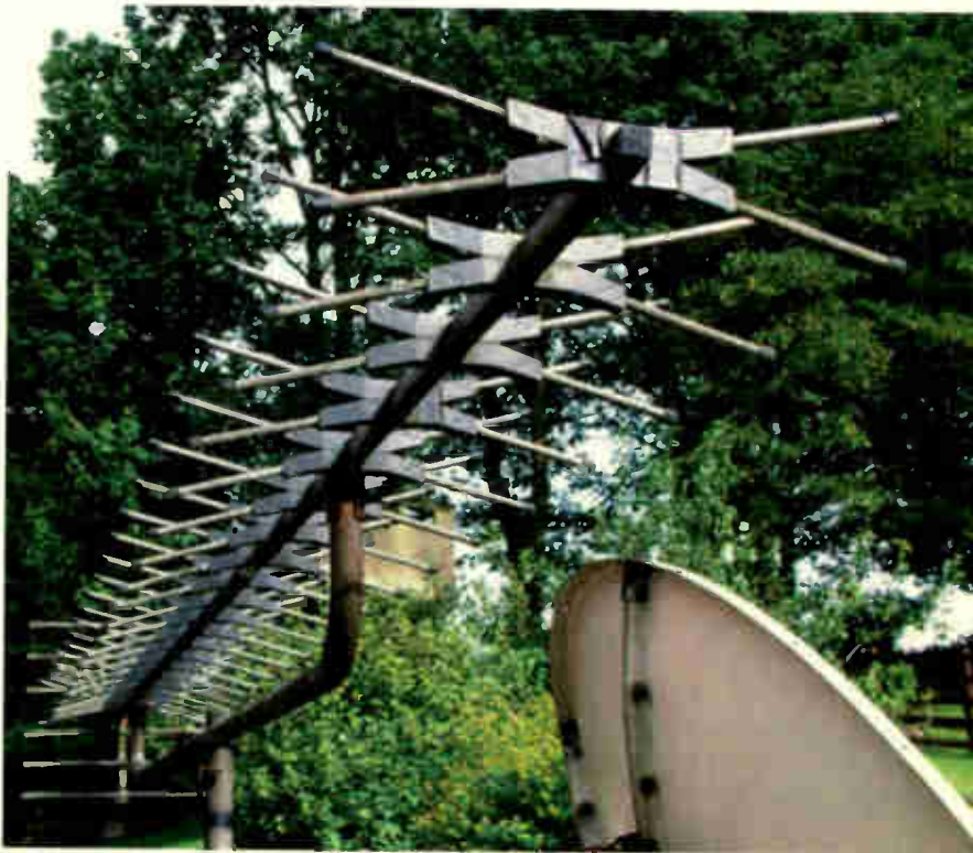
Bill Wright's Antiference XG21CD array critically mounted for reception from the Winter Hill transmitter in South Yorkshire.
