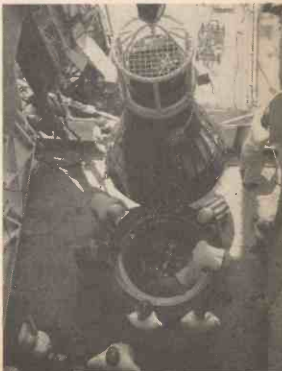
Mating of a Mercury Capsule to an Atlas vehicle.
