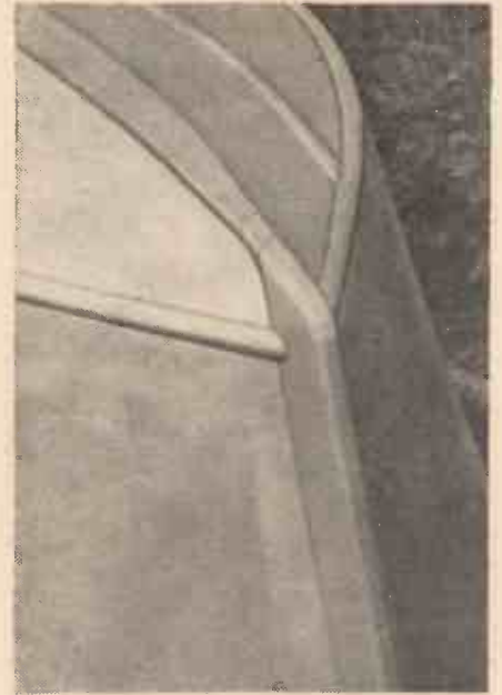
Fig. 15.—The finished cutwater.
