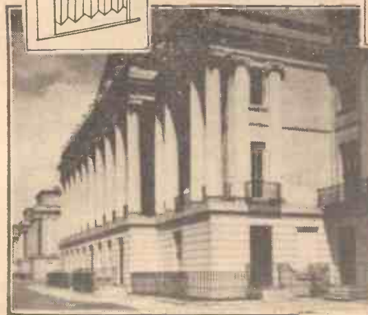
Fig. 3.—Using the rising front and swing back in order to obviate the necessity for tilting the camera. On the right is shown the sloping verticals which are the result of tilting the camera upwards.
