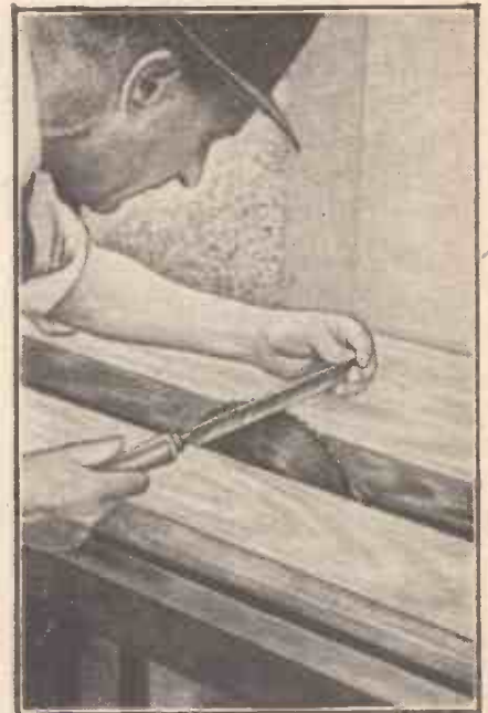
Fig. 6.—Touching up the blade in the bench.
