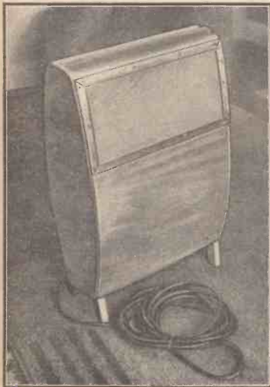
Fig. 2.—The completed heater.
