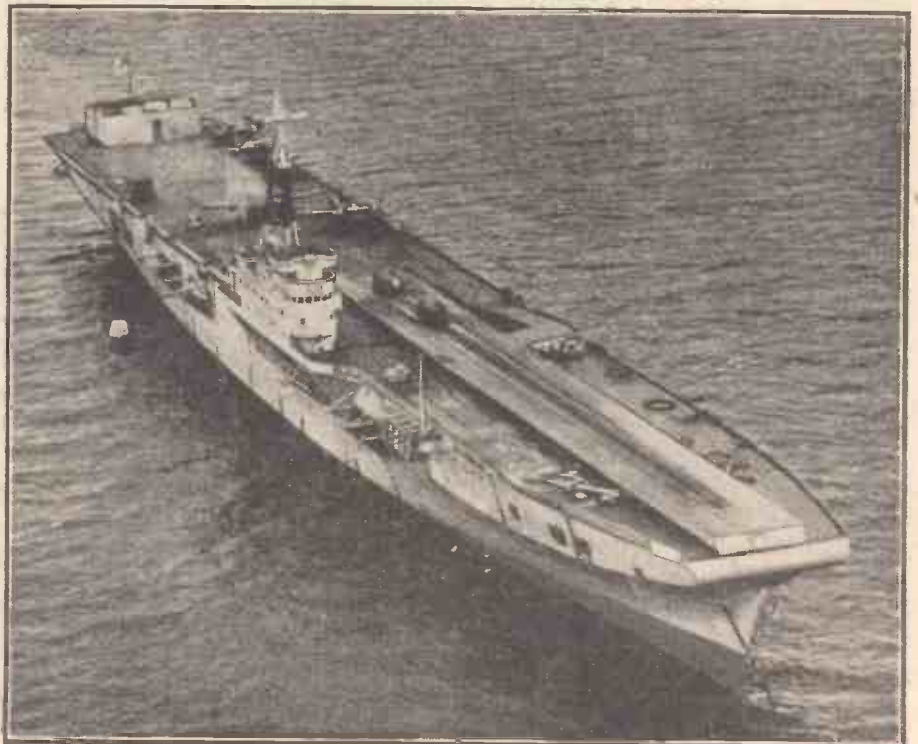
An aerial view of H.M.S. "Perseus," showing the steam catapult, which was installed in this ship for trials in 1951.
