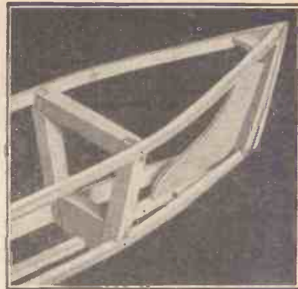
A general view of the bow construction.
