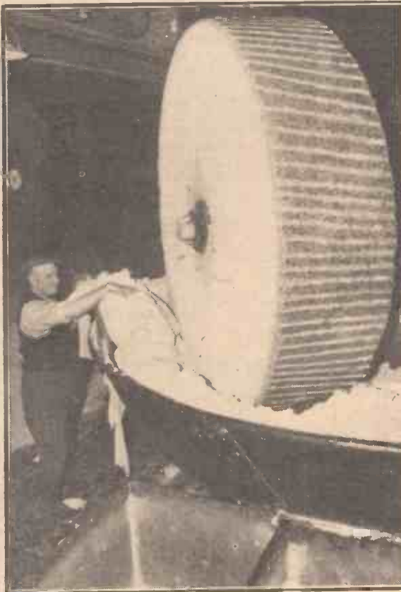
A large grinding stone used for disintegrating waste paper at the mills on the River Esk, in Scotland.
