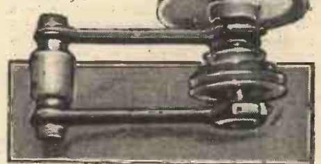
An improvised countershaft.
