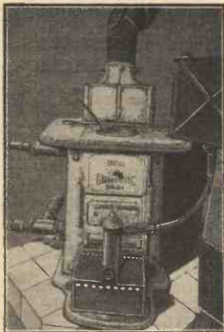
A burner using sump oil, fitted to a domestic boiler. Note. The water drip is not shown.
