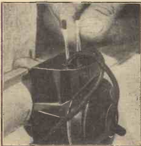
Holding wires in a plug socket with aid of matches is a common but dangerous practice.
