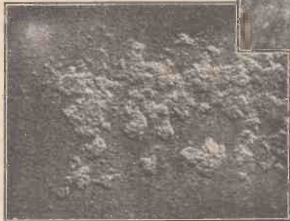
(Above) A surface photograph of newly quarried sandstone. (Left) Surface scales on sandstone. Unsightly and destructive efflorescences caused by the collection of soluble salt deposits on the stonework.
