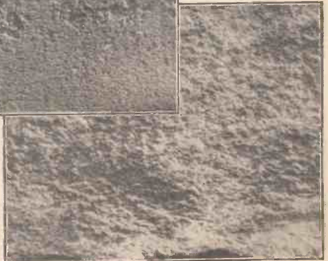
(Above) Stage 3, where the salt crusts on the stone surface have flaked away, leaving serious pittings and indentations on the stonework.
