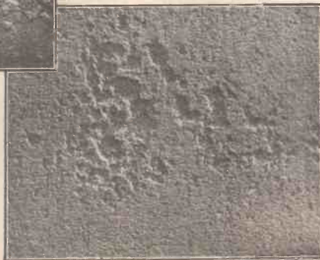
(Above) Stage 3, where the salt crusts on the stone surface have flaked away, leaving serious pittings and indentations on the stonework.
