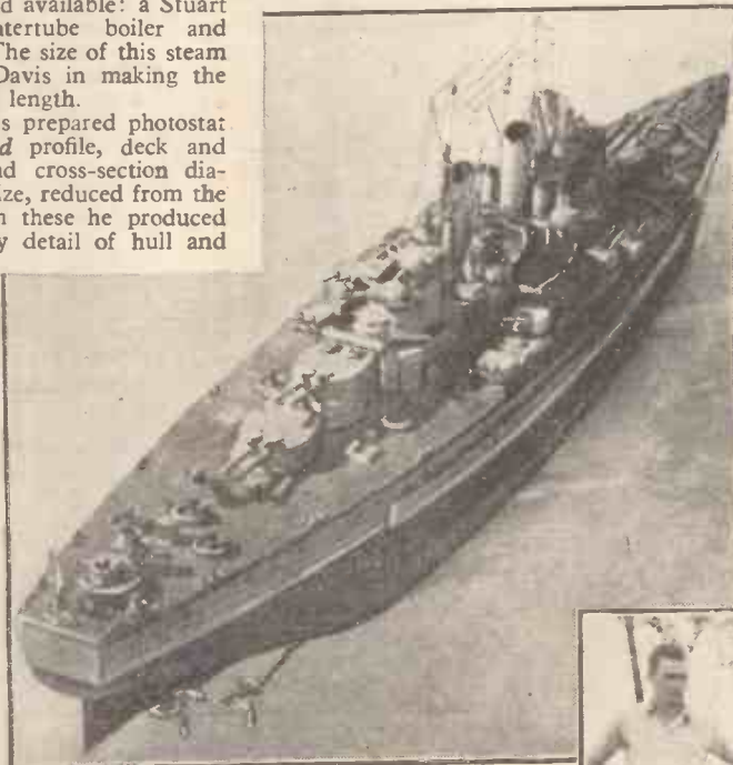
Fig. 1.—(Above) Mr. G. H. Davis's steam-powered model of H.M.S. "Vanguard," 5ft. long. All fittings for this model were made by the constructor.
