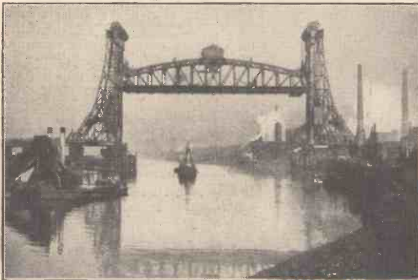
Fig. 13.—Tees (Newport) Bridge.—Dorman Long and Co.
