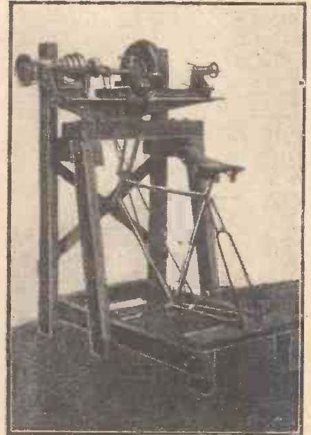
General view of the lathe stand and pedal driving arrangement.
