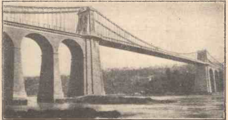
Fig. 9.—Menai Suspension Bridge.—Dorman Long and Co.
