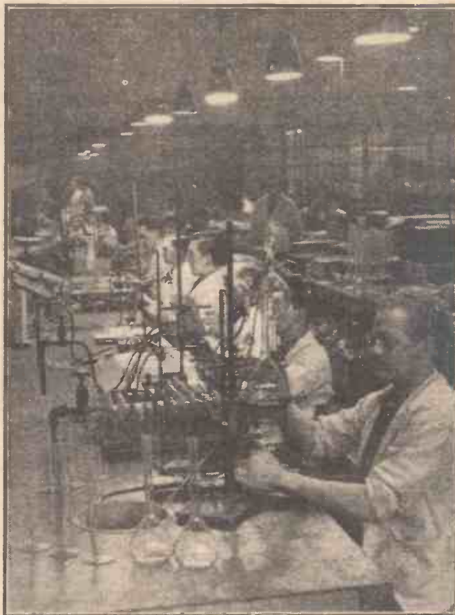
Calibrating scientific glassware to N.P.L. standards.
