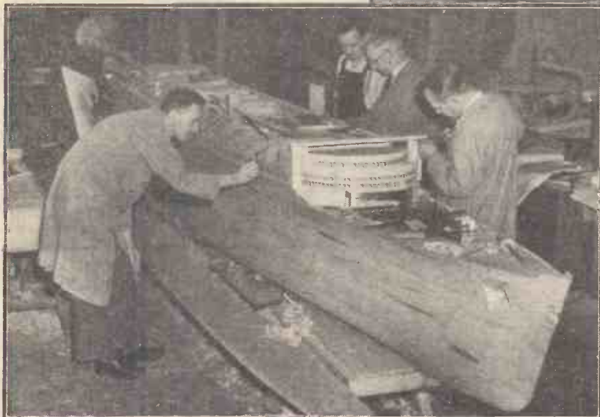
Fig. 4.—The first fitting of the superstructure.
