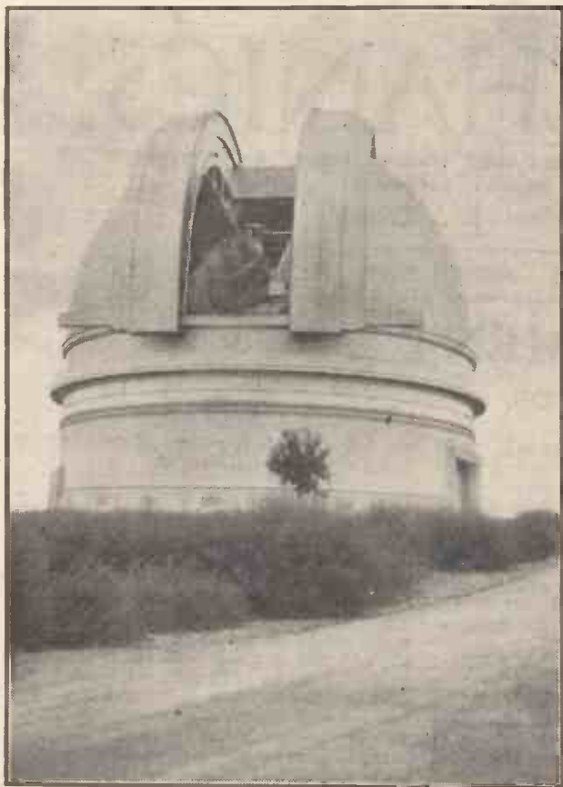
The observatory building, showing dome partially opened revealing the 200-inch telescope. The dome, which revolves on a circular track, is 137 feet in diameter and 135 feet high, and has a total weight of 1,000 tons.
