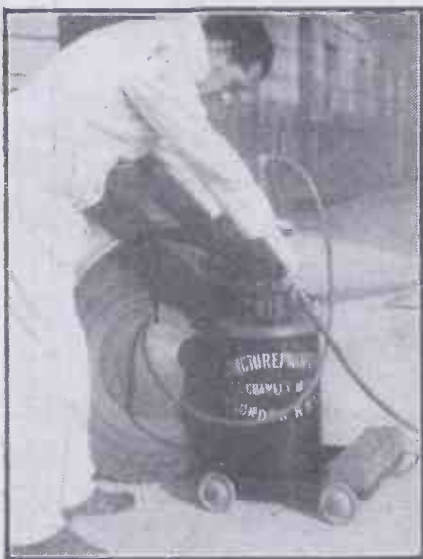
Pumping the Punctureprufe compound into a tyre.
