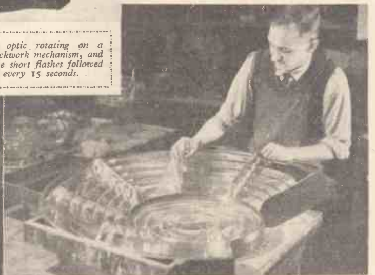
(Above) The finishing process after the glass prisms have been focused in the framework. This lens-panel is for the revolving optic of the Longstone Lighthouse. (Left) Grinding a glass prism so that it may fit into the lens framework inside a lighthouse lantern.
