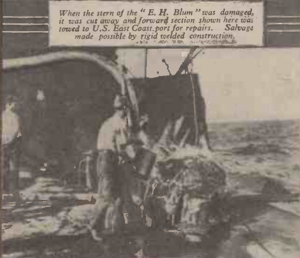
(Above) Crew of this disabled ship prevent fire from spreading by pouring water on oil tank covers. Note warped deck with weld seams still intact. (U.S. Maritime Commission photo, courtesy The Lincoln Electric Company, Ltd., Welwyn Garden City.)
