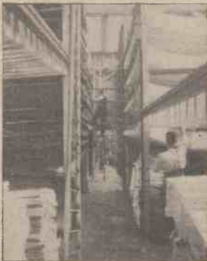
The conditioning room. Hanging up the finished hand-made paper to condition and mature under the influence of controlled humidity and temperature.
