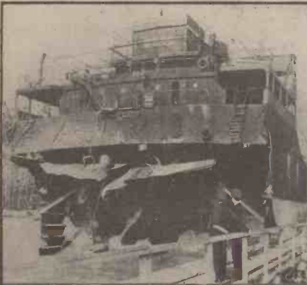
When the stern of the "E. H. Blum" was damaged, it was cut away and forward section shown here was towed to U.S. East Coast port for repairs. Salvage made possible by rigid welded construction.
