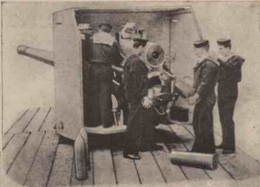
A 6in. quick-firing Elswick gun, designed for separate loading.
