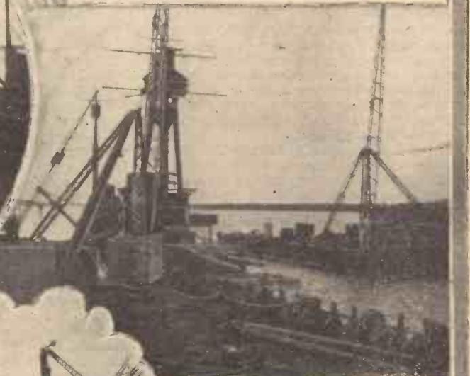
(Above) Showing a partly raised warship between the huge floating docks used in the operation.
