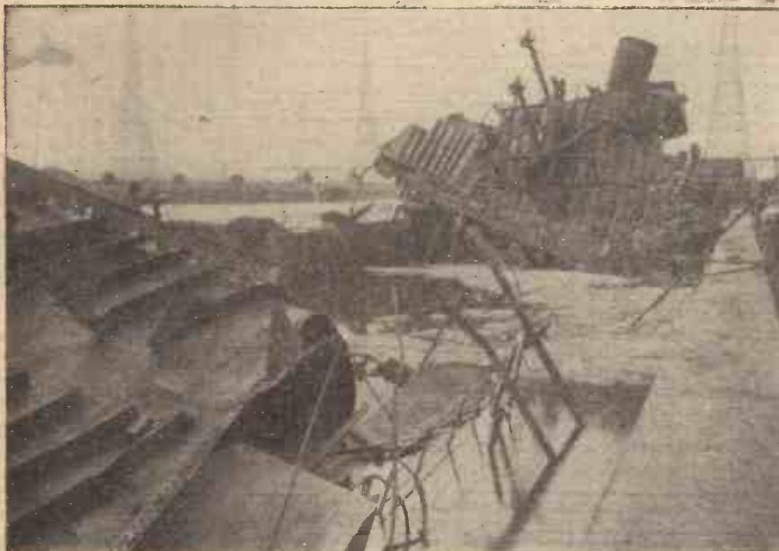
View of the S.S. "Liseta" looking aft, showing the deck rolled back in both directions. (By courtesy of the Anglo-Saxon Petroleum Co., Ltd.)
