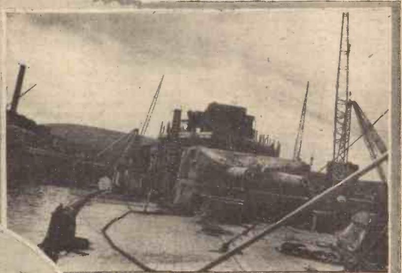
(Left) This illustration shows water being forced out of the partly raised hulk by compressed air.
