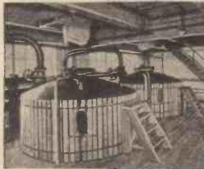
Modern extraction plant for the manufacture of strychnine.
