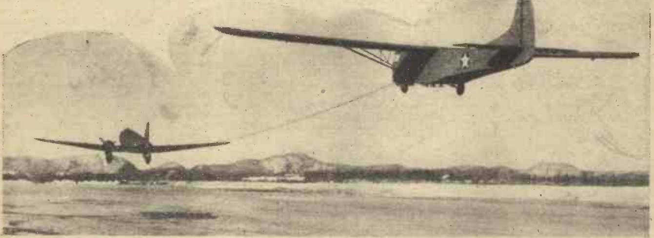
A troop-carrying glider, with a jeep on board, being towed by a transport plane.
