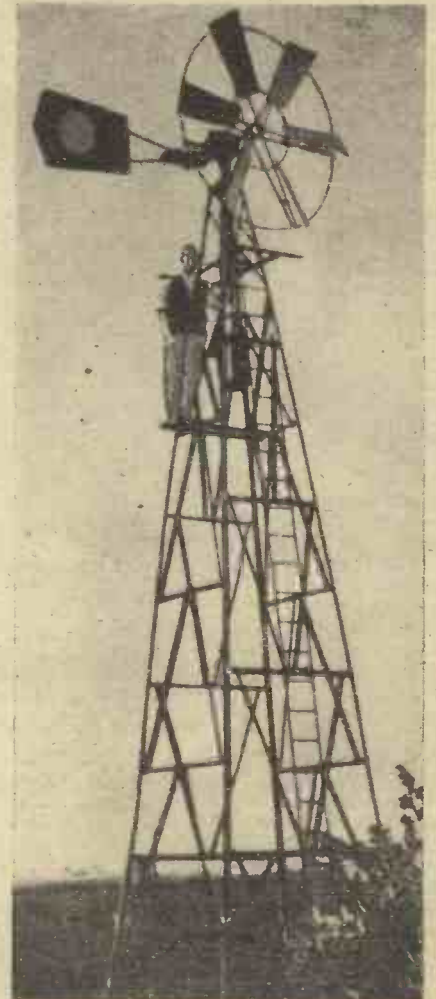
Fig. 2.—The finished windmill, with the owner aloft.
