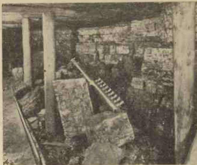
Fig. 4.—After the bursting has taken place, showing the manner in which the coal is brought down. Note the size of the lumps brought down and the pistons now fully extended.
