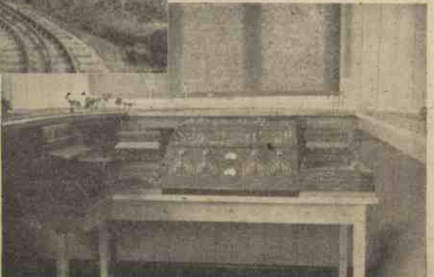
Westport-Seaview Branch, L.M.S./G.W. Joint Line. Control panels: 1, controller, Westport station; 2, controller, Westport goods yard; 3, controller, main line; 4, controller, Seaview station. Signal lever frames interlocked. Signal cabins are replicas of large frames.
