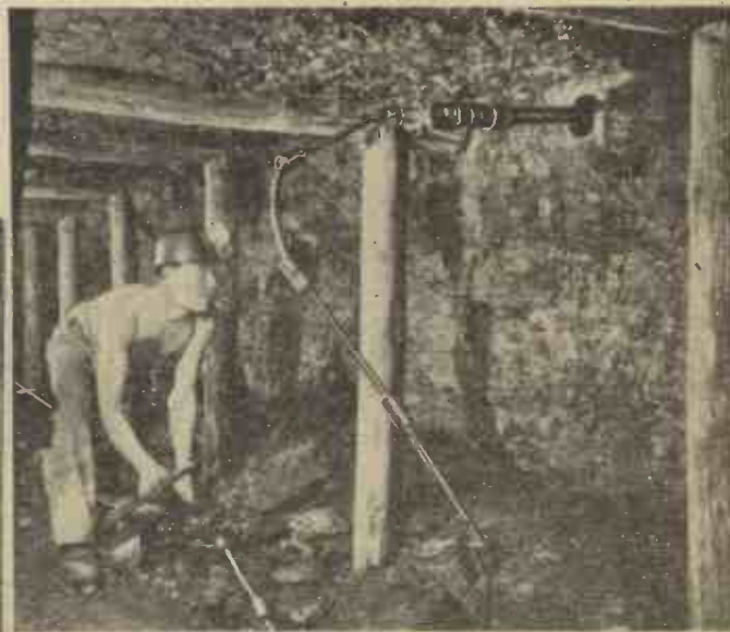
Fig. 3.—Building up pressure by means of a hand pump.
