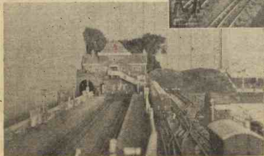
Another view on Colonel Stewart Law's No. 3 railway. Seaview Station, a residential seaside resort with busy daily business traffic from Westport (single line).
