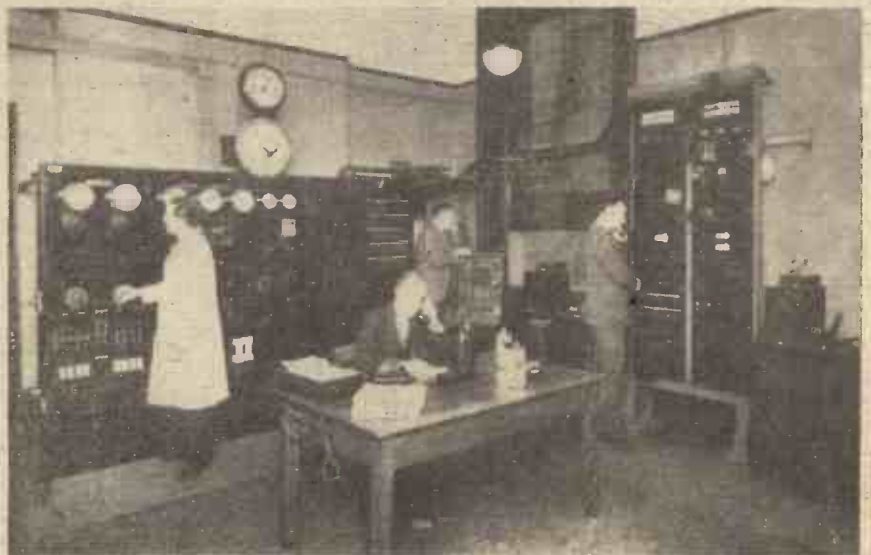
The Picture Telegraphy Department of the Central Telegraph Office. The power switch-board is on the left, and the control panel on the right. (By the courtesy of the Postmaster-General.)
