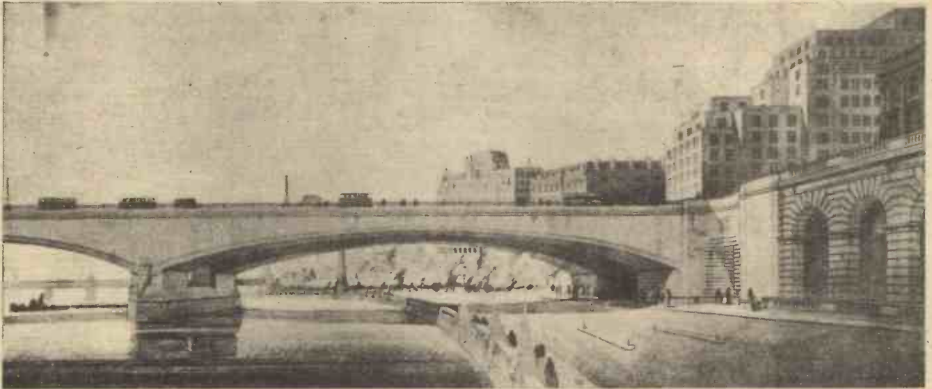
A drawing of the northern end of the bridge, showing how the first arch spans the Embankment. (By the courtesy of L.C.C.)
