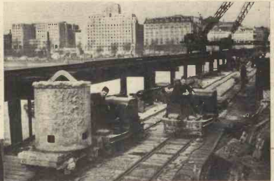
(Above) A skip loaded with 1½ tons of concrete being drawn along on an electric truck.
