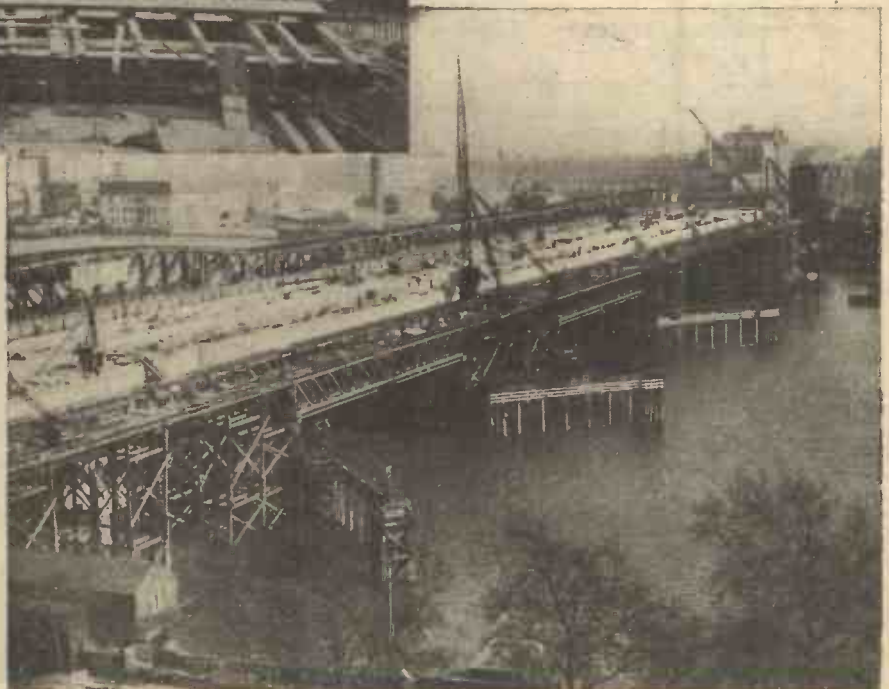
Placing the massive reinforced concrete girders in position. (Right) The new bridge nearing completion. Note the service gantry, with its cranes, from which the bridge was built.
