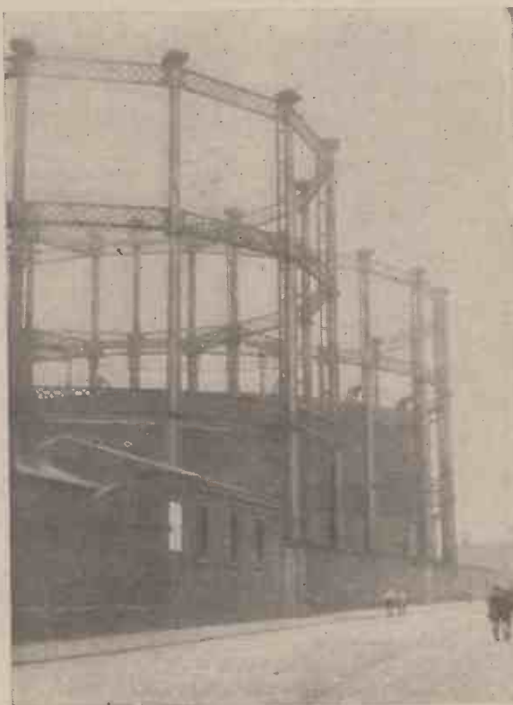
From William Murdock's pioneer gas lighting experiments the enormous present-day gas-producing industry has directly descended. Here is a pair of modern gas-holders, each containing thousands of cubic feet of coal gas.
