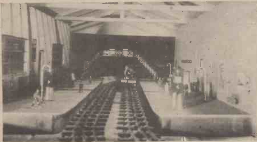
The interior of the "greenhouse" station, with express entering, hauled by L.M.S. Compound.
