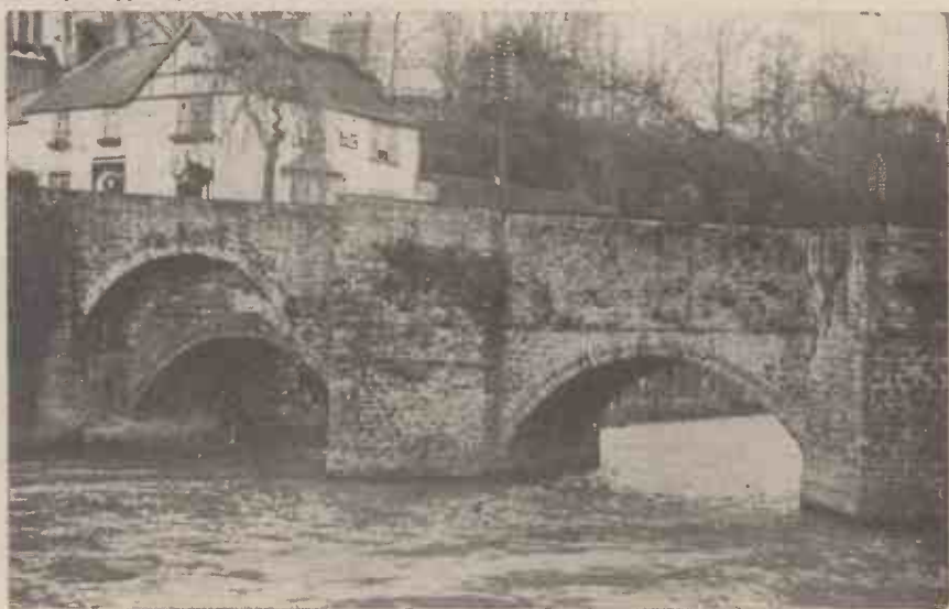
Ludlow Bridge across the Teme, Ludlow.
