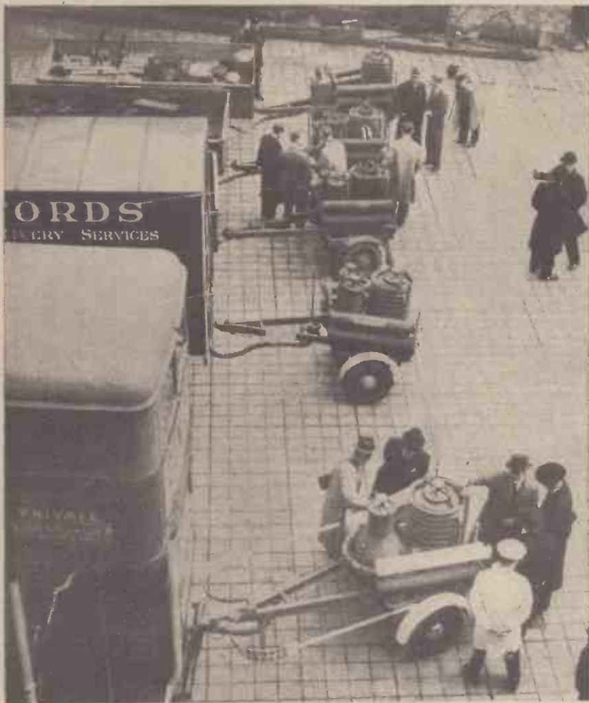
Producer-gas vehicles attached to various types of vehicle
