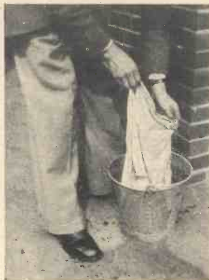
Canvas soaked in a solution of copper sulphate is rendered rot and mould proof.
