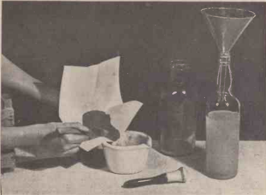
The dried pigment is placed into a mortar for grinding.
