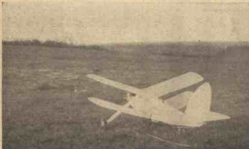
Fig. 3.—A very small landplane with biplane arrangement of lifting surfaces.
