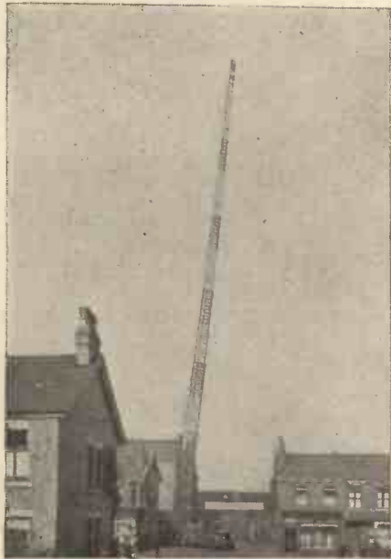
A fire escape capable of 180 ft. vertical elevation in the air designed by the Leyland Motor Company. An escape of such dimensions was found necessary owing to the rise in height line of modern buildings.
