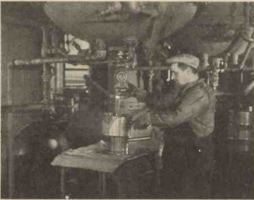
One of the stages in the casting of phenolin cast resin-catalin.
