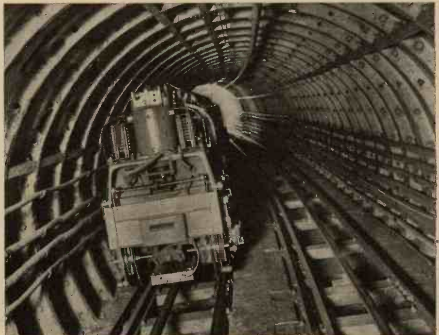
Showing a train passing along one of the many tunnels.
