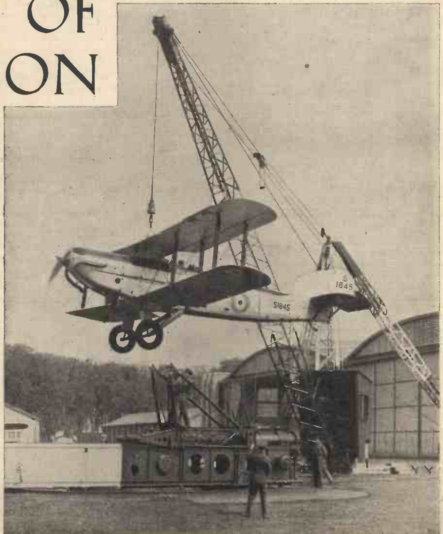
One of the most striking features of the Empire Air Day display at the Leuchars Aerodrome, Fife, recently, was the catapulting into the air by means of a cordite charge, of a Fairey machine. The catapult was the only one of its kind on view in Britain, and is similar to that used on battleships.
