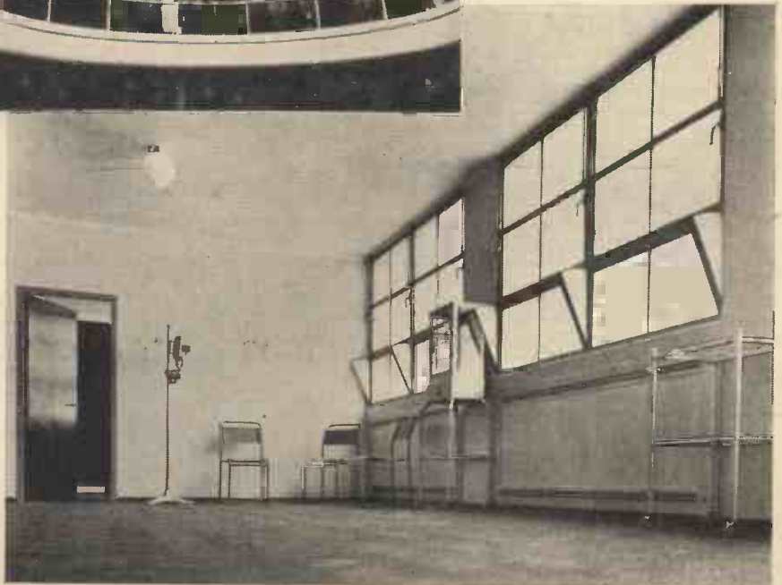
(Top Centre) The laylight of a London store glazed with Thermolux, a new kind of glass which eliminates all shadows, at the same time preventing rooms glazed with it from becoming too hot in summer and too cold in winter. (Below) Showing the use of Thermolux in the new tuberculosis dispensary at Devonport Street, Stepney, E.
