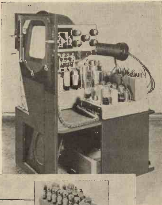
The G.E.C. television receiver removed from its cabinet. The double time-base is in the foreground.
