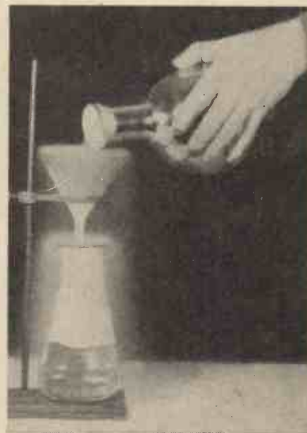
Liquid air being poured from one vessel to another. Note the ring of frost around the edge of the upper vessel.
