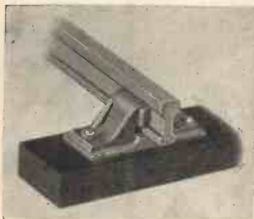
Actual Photograph of Bond's British Permanent Way.
