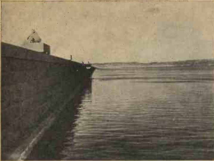
The Aswan Dam, showing the water held above it. The height of the Dam at first was 130 ft., but it has since been raised 17 ft., and the thickness doubled.
