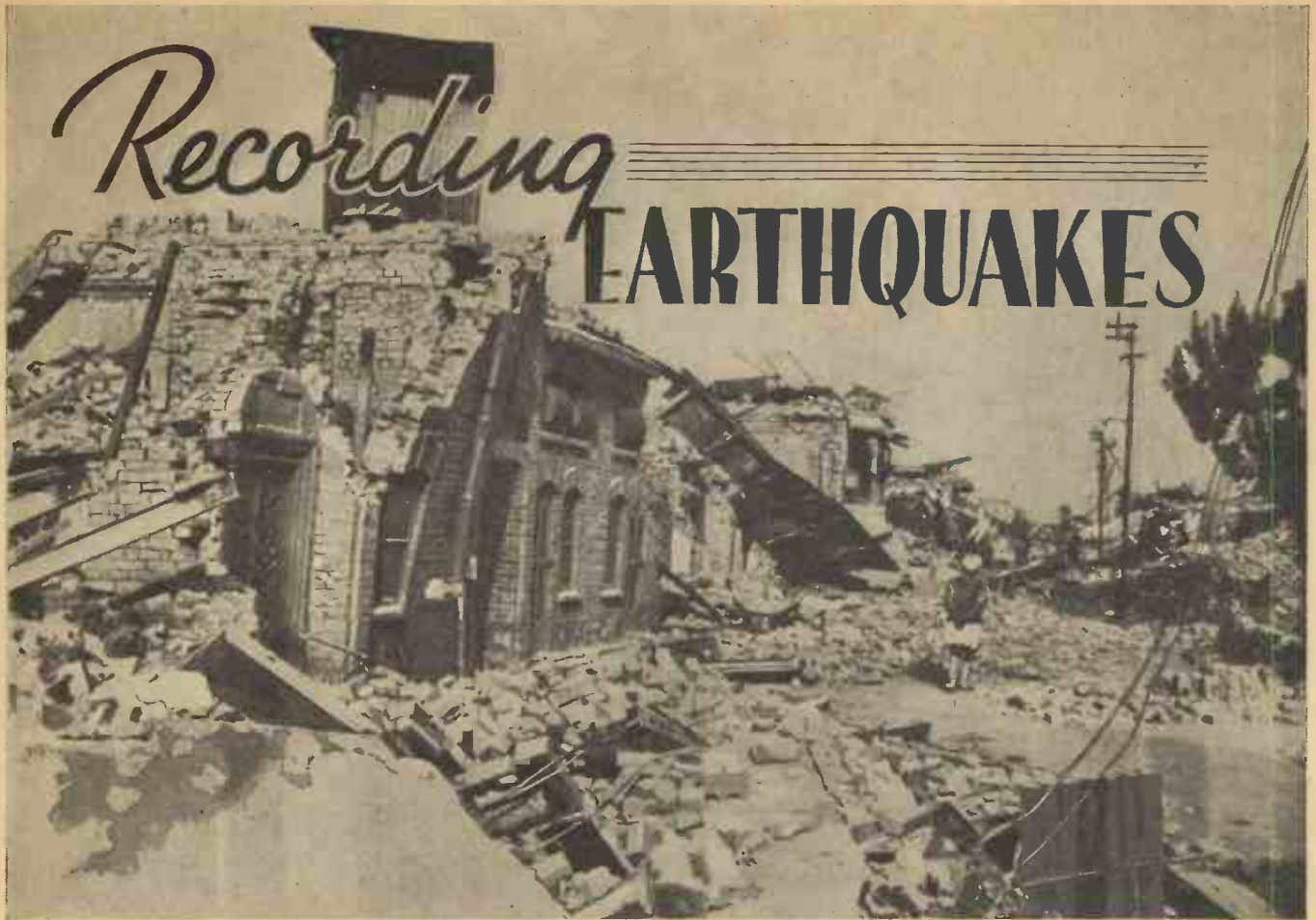
Fig. 1.—A view of a street in Quetta after the earthquake in May last year when over 30,000 persons were killed.
