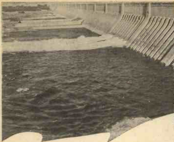
The Dam showing the sluices, only a few of which are working.
