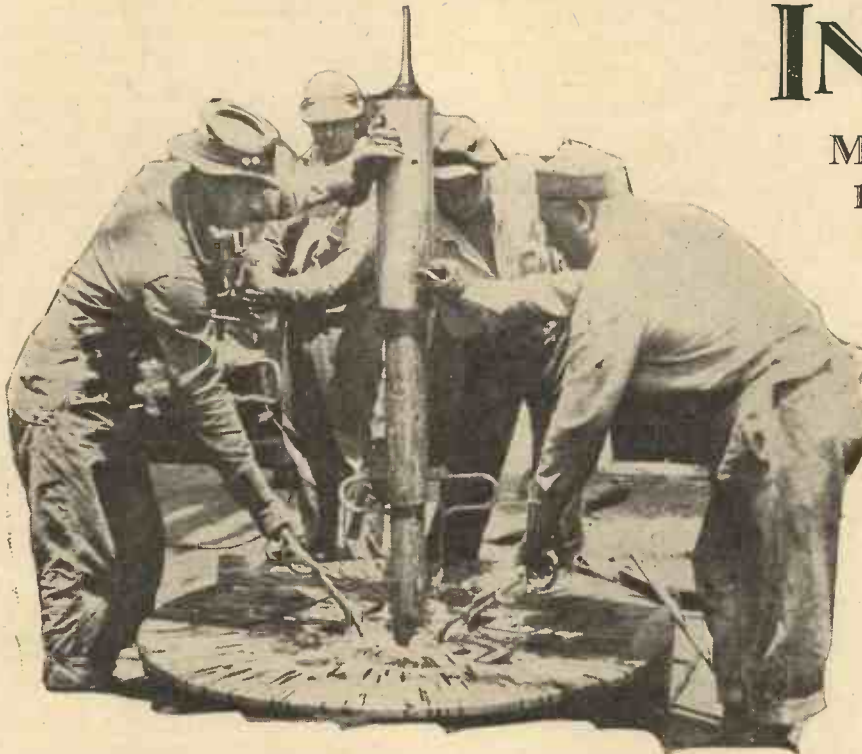
Considered to be the deepest hole in the world, this shaft was sunk by the Shell Oil Co. at Signal Hills, near Long Beach. The illustration shows workmen removing the bit with the valuable geological specimens it brings to the earth's surface.
