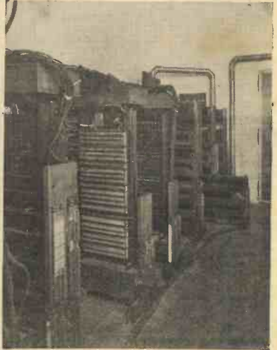
Action relays and switch boards, in course of construction.
