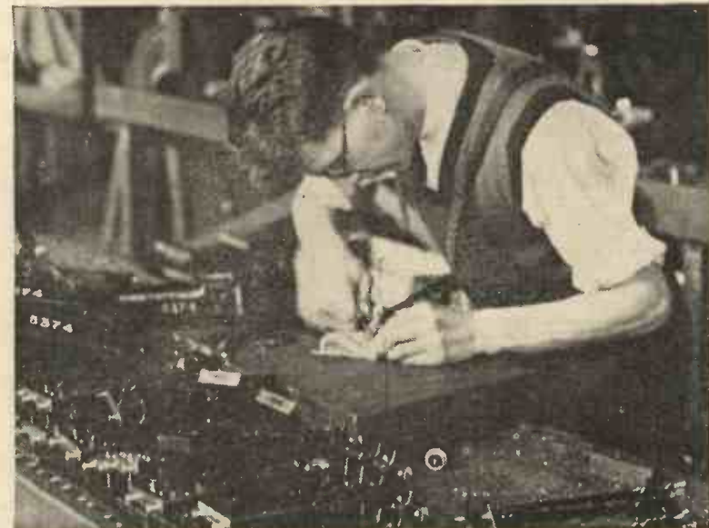
Fig. 3.—A part of the assembling table—fixing the buffers and buffer beams to the under-framing.
