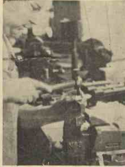
Fig. 4.—Assembling the cylinders.
