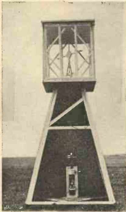
By means of two lighthouses similar to the one shown, emitting "light waves," it is possible to acquaint the pilots of aeroplanes of dangerous atmospheric areas and to point out the safest route to follow.
